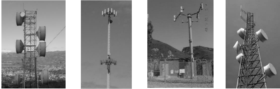
Examples of Non-Stealth Wireless Communication Facilities
