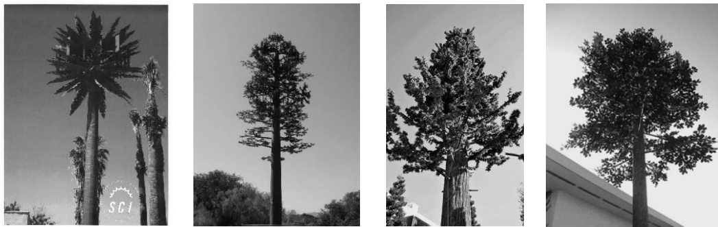
Examples of Faux Trees (Wireless Communication Facilities)
